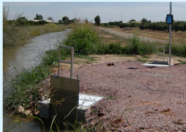
Figure 4: A completed MACE AgriFlo meter outlet. Head ditch is to the left.
