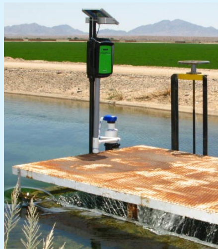
Figure 1: The broad-crested weir structure at Quail Mesa Ranch, AZ.
