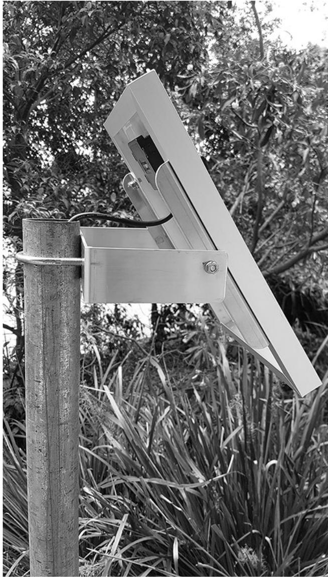
11. The cables from the solar panel/charger to the electronics unit must be enclosed to minimise exposure to the elements. The cable should be either routed through conduit or through the solar panel mounting pole. You will need a hole drilled in the mounting pole at the top near the solar panel as well as a cut away where the electronics unit is to be mounted.
