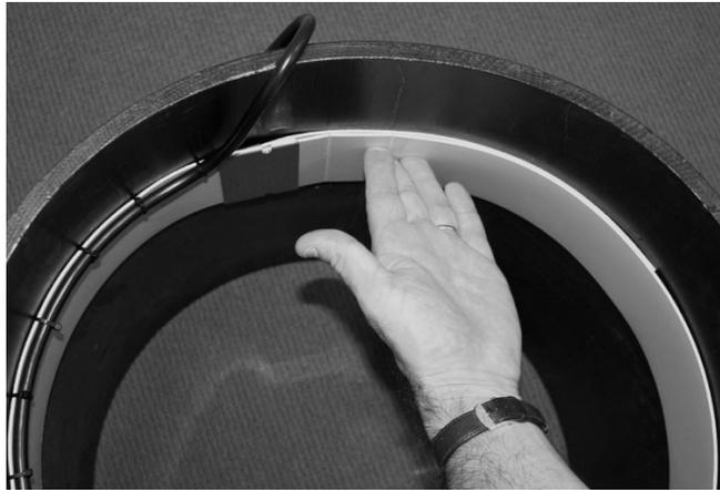
13. Carefully route the cable from the sensor back to where the XCi device enclosure will be mounted.
