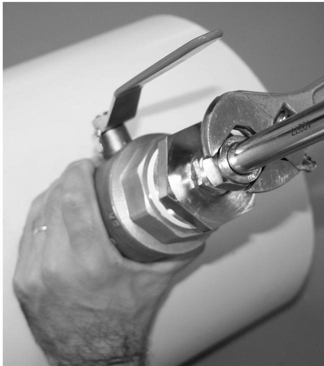
13. When the installation is complete, the sensor shaft should be pointing directly towards the centre of the pipe in all planes.
