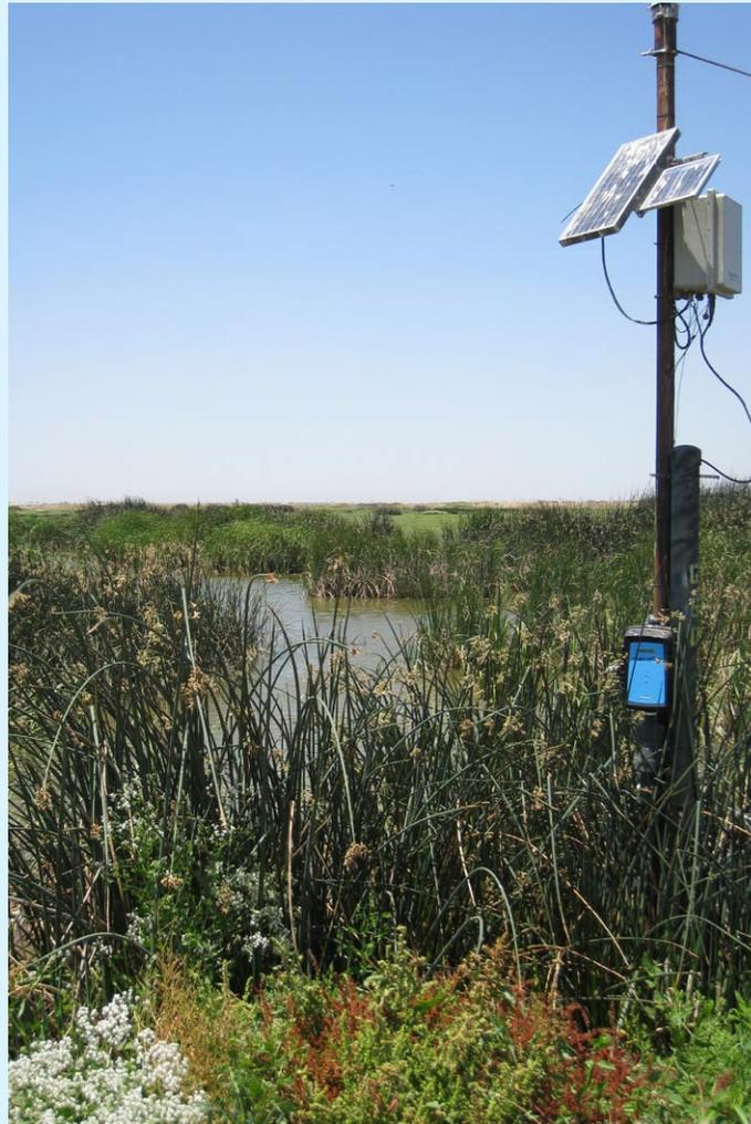
Figure 3: A Series3 AgriFlo installed on the outlet of a lagoon.
